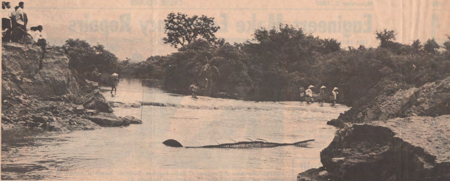
FLOATING CULVERT —The Son Cai River carries a piece of floating culvert—evidence of the destructive power it can possess when stirred by monsoon rains.
