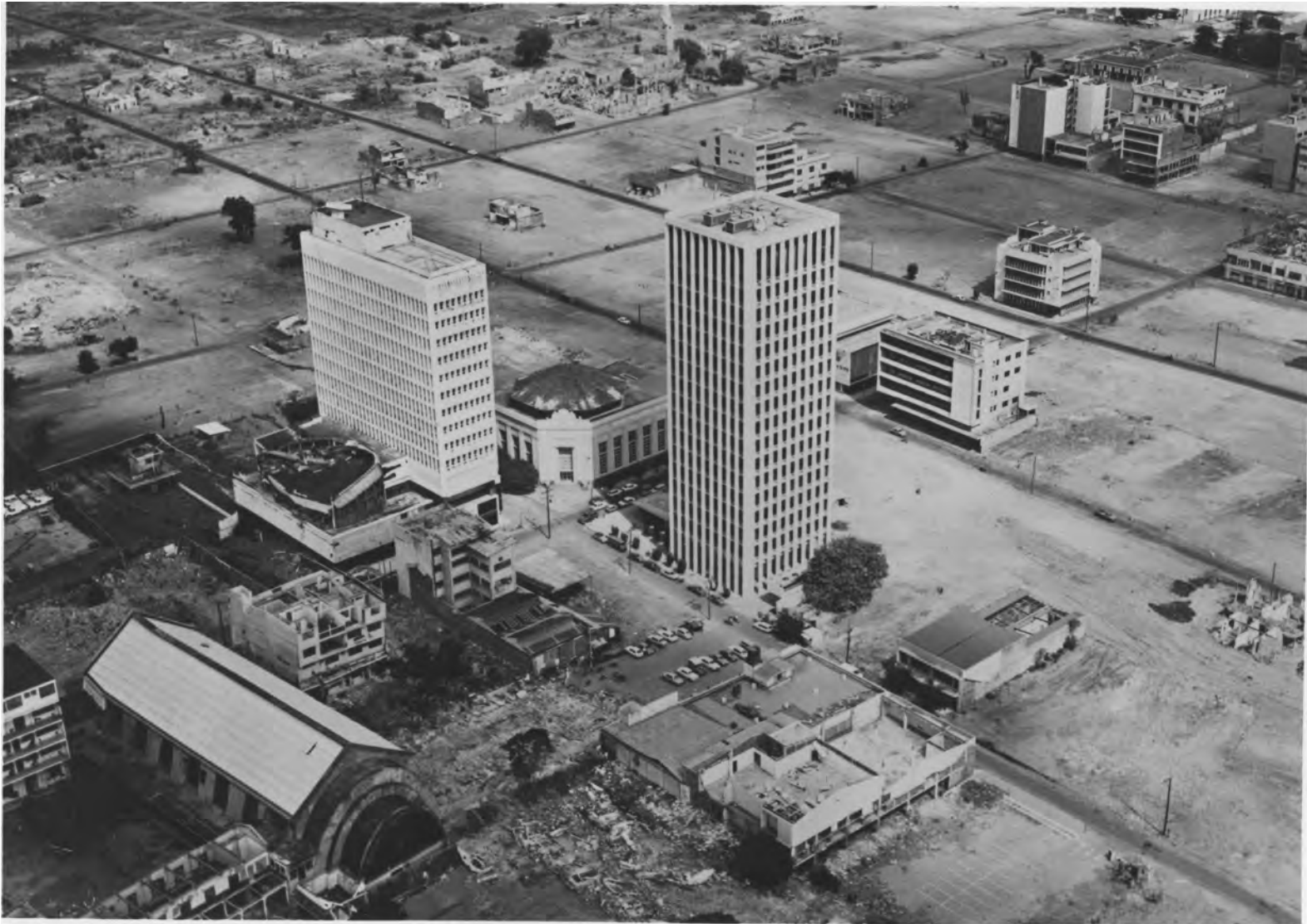
Downtown Managua in March 1974 after debris has been removed. The Central Bank building (left) must be reduced to two or three floors, because of structural faults. Other buildings, such as the one to the right of the Banco de America tower (center), have been razed.
