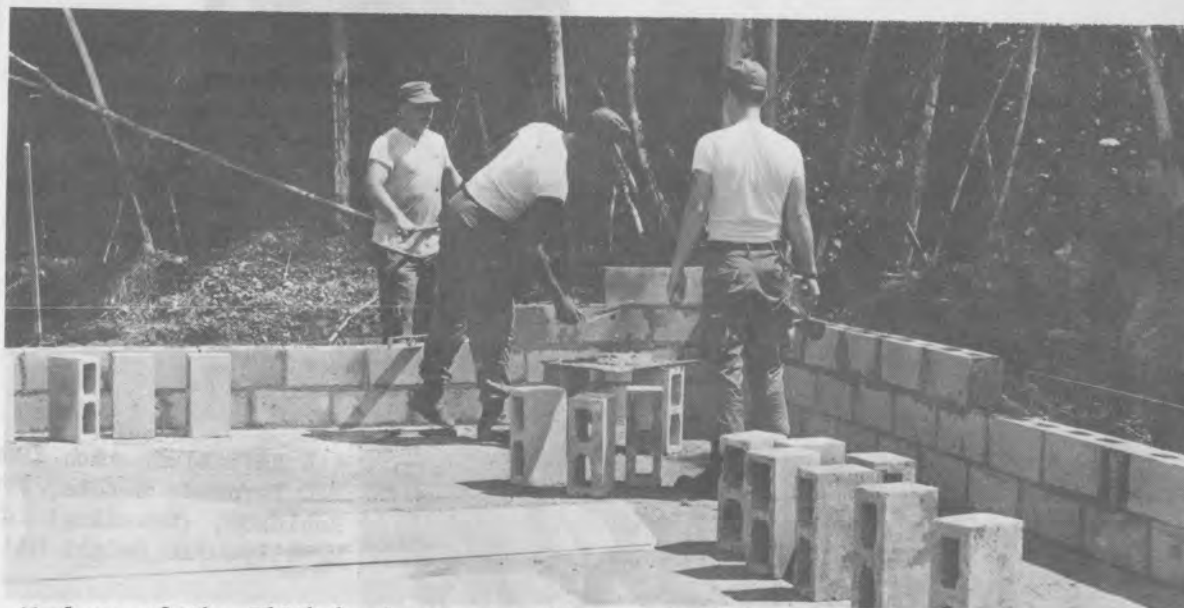
Members of the 518th begin construction on building.
