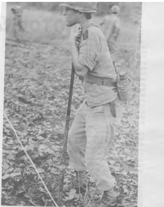
SGT Pedro Saenz, Jr., uses pole to punch borehole for dynamite to be placed. The entire area was under standing water. (Note mud on the pole).
